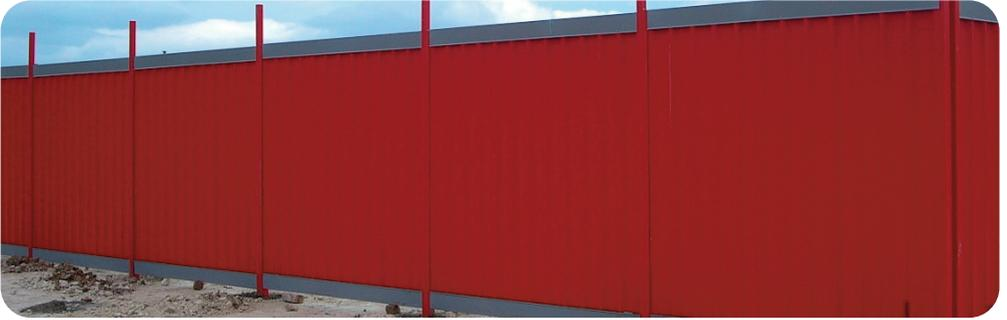
Fortress™ is our 2.4m steel in-ground site hoarding widely used on construction sites throughout the UK and Ireland where a robust steel perimeter or site compound is required. Fortress™ is available with a variety of door and gate
