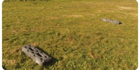
Place the second rubber block the required distance from the first block. Continue this process along the entire length of your intended fence line.
