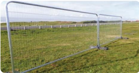
Insert the first and second fence panels into the first three blocks (centre holes) and connect with two couplers and tighten to 7NM or 5lb/ft. Repeat until installation is complete.
