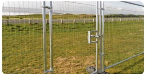
The latch pole should be placed in the next block and connected to the next panel in the fence line, ensuring the catch is lined up with the latch of the gate.
