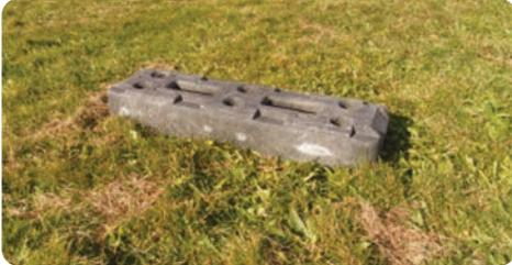
Place the first rubber block at the proposed starting point of the fence line.
