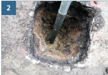
2 Excavate holes to required dimensions and set scaffold tubes in place using concrete (ensure tubes are upright and level).
