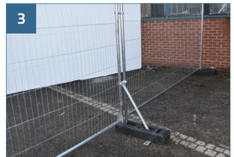
Attach nut and tighten (recommended torque 13NM) to secure brace. Repeat along fence line until installation is complete.
