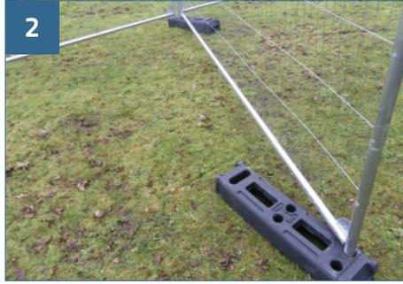
2 Insert a mesh panel into the round hole farthest away from the fence line as shown.
