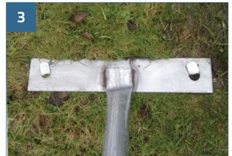
Insert support brace pegs through holes in base plate using appropriate tool, and repeat steps 1 to 3 along the fence line (please note that you should scan for services where pegs are to be placed).
