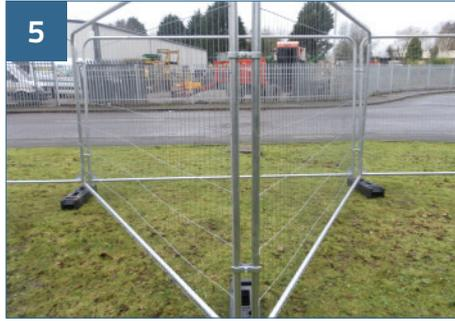
5 Connect both panels together using two couplers as shown and tighten (recommended torque 13NM).
