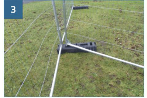
3 Insert the other end of the panel into the rectangular hole closest to the fence line as shown.
