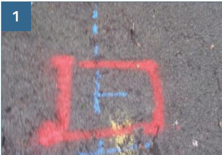
1 Mark the positions of the holes for the scaffold tubes at the required distance apart along your intended fence line (use 2 scaffold tubes for the 1st and last panels).
