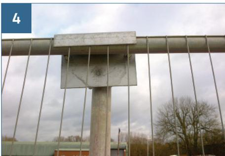
4 Connect the top BK clamps, as shown, and secure top of the panel by tightening bolts (recommended torque 13NM) ensuring the panel is level.
