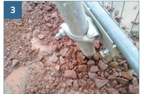
3 Offer the first panel up to the first tubes and connect the bottom BK clamps in place, as shown and secure bottom of panel by tightening bolts (recommended torque 7NM—5lb/ft).
