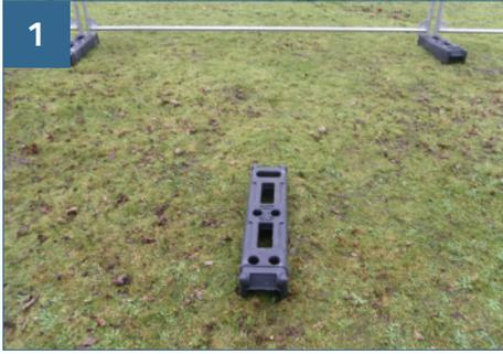
1 Place a rubber block mid point at the required distance in line with the first panel to be braced, as shown.
