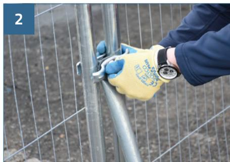
Continue normal installation, placing the panel in front hole. Now remove the nut from one coupler and attach brace as shown.
