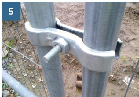
5 Place the next panel in position and connect to the first panel using two couplers as shown. Re-repeat steps 3 and 4.
