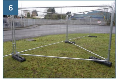
6 Connect both panels to the fence line using the same method as in step 5, as shown. Repeat at required intervals along the fence line until the installation is complete.
