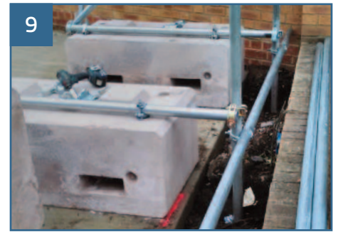
9 Connect your first 10ft horizontal rail at the bottom of the vertical frames using Single Scaffold Fittings, as shown.
