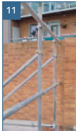
11 Once the bottom rail is fitted, repeat steps 9 and 10 for the middle and top rails. Placement is to suit your hoarding height.
