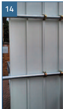
14 Fit the next board into position and slot into the first board. Connect the board joint to the horizontal rails, using Go Hoard clamps, as shown.
