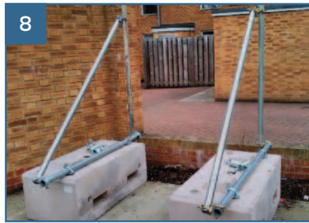
8 Repeat steps 3 to 7 on all blocks along your intended hoarding line.
