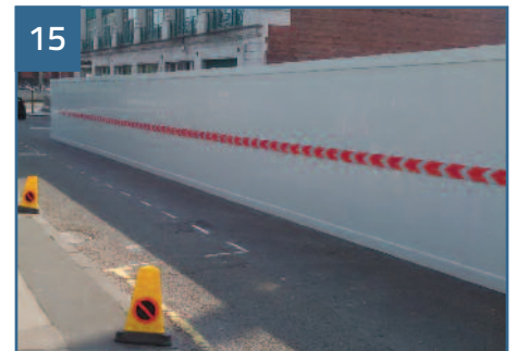
15 Repeat step 14 until all boards are secured along the entire hoarding line.
