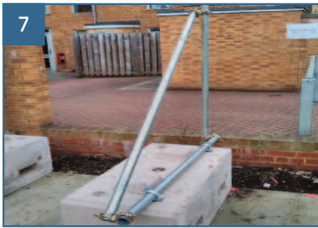
7 Connect the other end of the 6ft tube to top end of the 8ft tube using another swivel fitting as shown and tighten all nuts.
