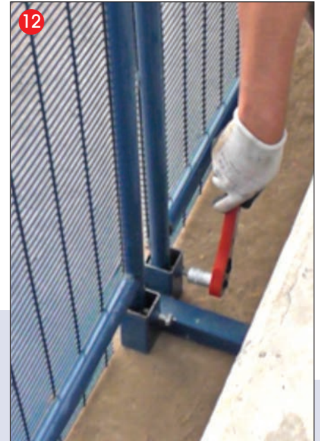
Tighten M10 captured bolt securely against Panel leg to prevent lifting. (Recommended Torque: 22N m, 16.2ft lb)
