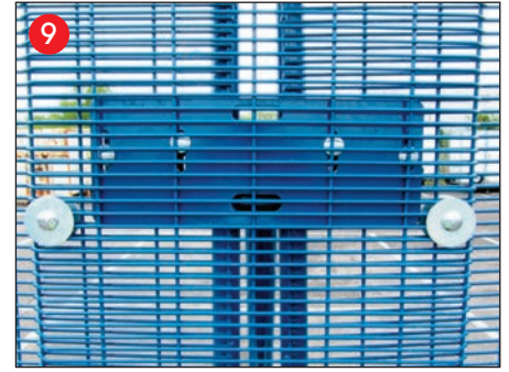
Attach Cover Mesh over Clamp Plate and Panel gap using M8x50 Coach Bolts with M12x50 washers (attack side), M8 Full Nuts and M8x50 washers (inside).
