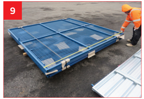
9 On level ground use the combined width of both gate leaves, plus 250mm.
