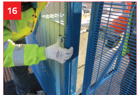
16 Attach adjacent Polmil Mesh Panels to front face of Gate Post using M8x150 Coach Bolt Set.
