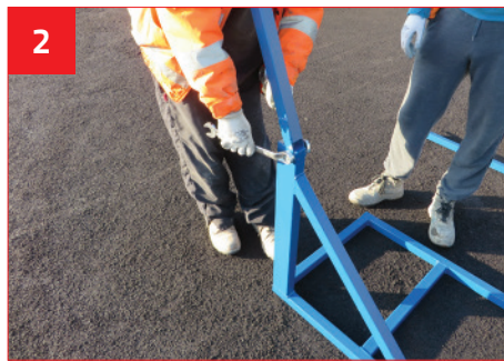
Attach Short Front Brace and Long Back Brace to Support Base with M16 Hex Bolt Set.
