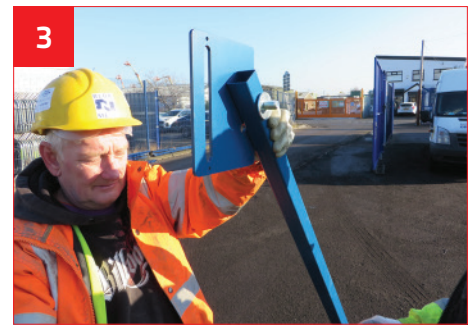
Attach Brace Plates with M16 Hex Bolt Set (On level ground use centre hole).
