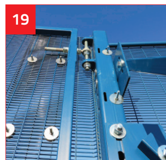
19 Bolt on optional Cover Mesh to protect Hinge gap.
