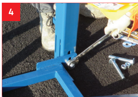
Attach bottom of Gate Post to Support Base with M16 Coach Bolt Set.
