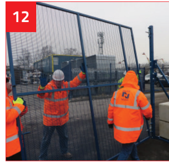
12 Slide Gate Leafs onto Hinge eye bolts.
