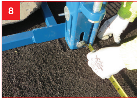
8 Check distance between Gate Post faces. See 'Top Tip' above.
