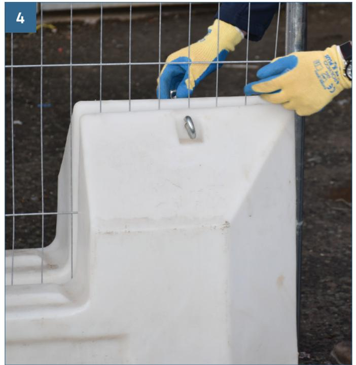
4 Replace nut and bolt and tighten to secure mesh panel (13NM).
