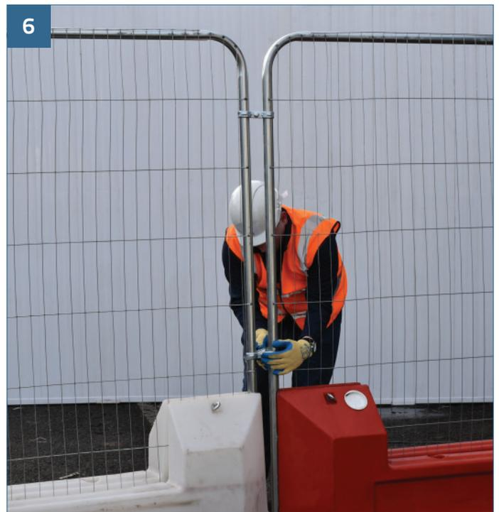
6 Repeat steps 1 to 5 along your intended installation line, connecting panels with couplers as shown and tighten (13NM).
